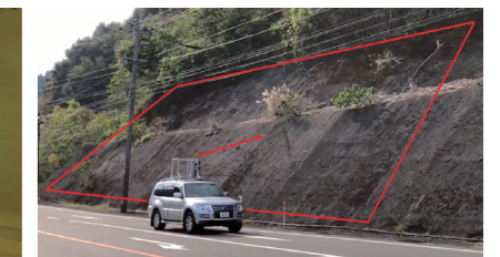
Image of slope surface
