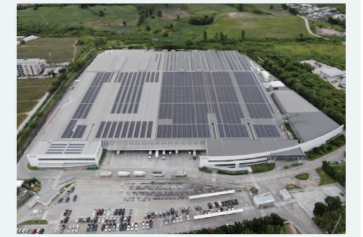
Roof of Ricoh Manufacturing (Thailand) Ltd. plant
