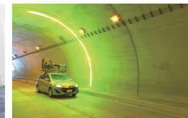
View of tunnel interior
