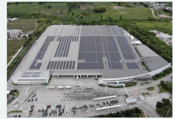
Roof of Ricoh Manufacturing (Thailand) Ltd. plant
